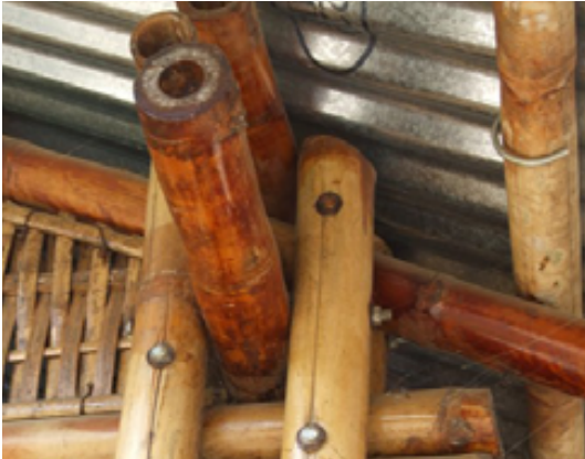
On the left: Bamboo column-beam-truss connection (photo: K. Harries). On the right: participants of the TC kick-off meeting, in hybrid mode, in Milan in April 2024 (photo: D. Ciancio).
