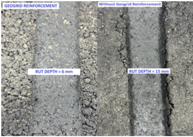
Top view geogrid-reinforced asphalt pavements and test results showed that the geogrid-reinforced pavements improved the rutting resistance by 50 % compared to unreinforced pavements ©Dr Lek haz Devulapalli; Ms Sreelakshmi S; and Dr Sreekumar TV Funding Agency - National Technical Textile Mission (NTTM), Ministry of Textiles, India
