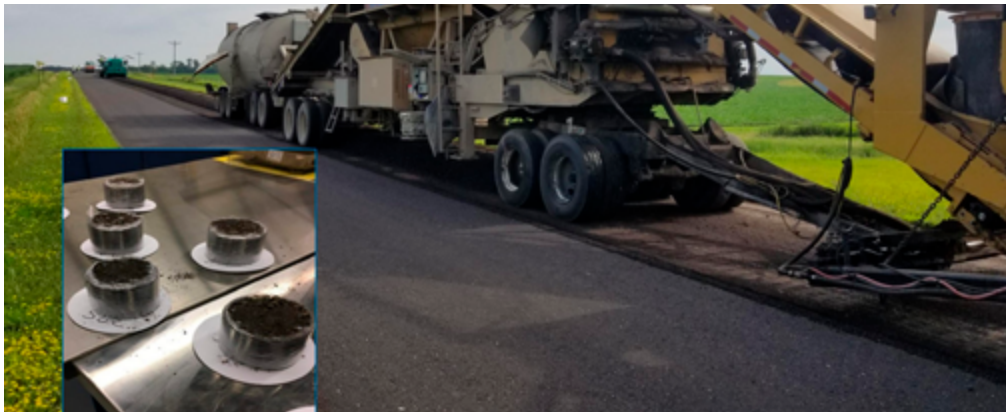
Cold recycling of asphalt pavement. Insert: Partially sealed drying of cold recycled asphalt specimen in lab that was part of the inter-laboratory testing effort of TC 264-RAP to improve laboratory curing procedures. Picture courtesy of A. Carter and E. Dave.
