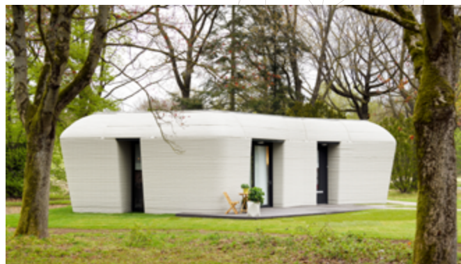
3D concrete printed house. Image courtesy of B. van Overbeeke.
