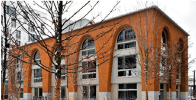
Rammed earth building in Lyon, France. Image courtesy of Erick Salliet. Architects: Clément Vergely; Structural Eng.: Batiserf; Contractor: Nicolas Meunier-Le pisé.
