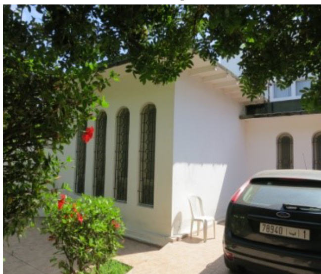
Fig. 1 – Experimental house made with Béton banché (walls and roof).
