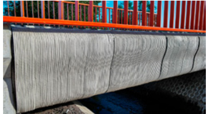
3D printed concrete bridge in Gemert, Holland. Courtesy of Marczoutendijk.
