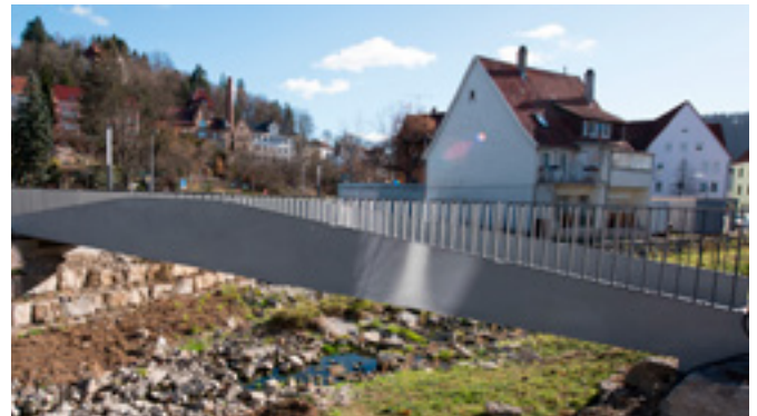
TRC bridge in Albstadt-Ebingen. Courtesy of Solidian.
