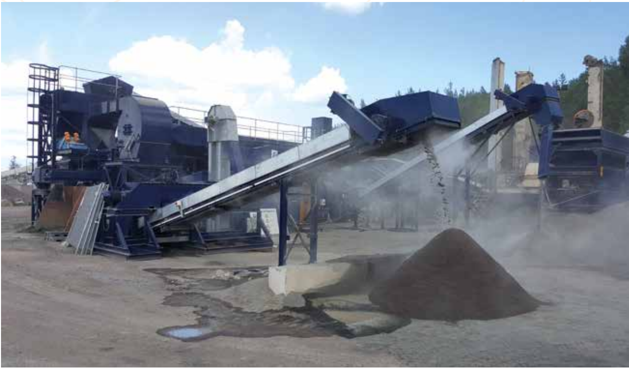
Test-production of crushed sand for concrete at a pilot-plant within the MiKS-project at the Norwegian University of Science and Technology. Credits: Roland Cepuritis and Stefan Jacobsen
