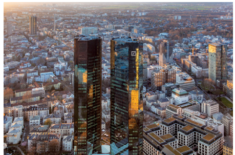
Deutsche Bank AG - Frankfurt am Main Core reinforcement using CFRP
