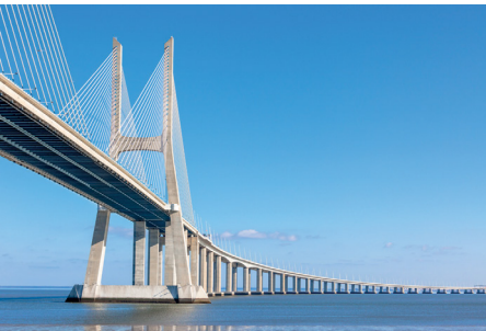
Vasco da Gama bridge - Lisbon Bridge columns reinforced using CFRP
