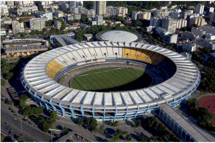
Maracanã Stadium - Rio de Janeiro Structural reinforcement using CFRP
