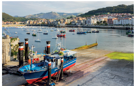
Paseo Marítimo – Castro Urdiales, Spain Structural repair using FX-70®
