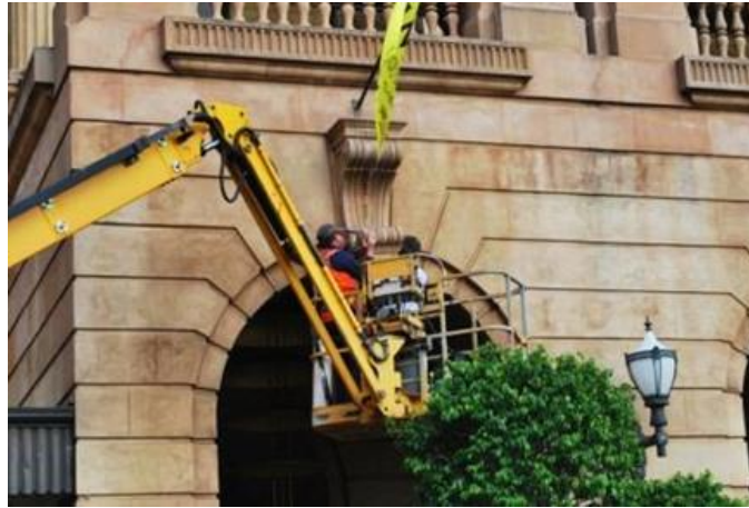
Figure 3. Removal of loose items.
