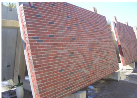
Pre-insulated thin brick precast panels
