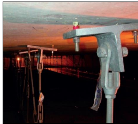
Figure 2. Concrete ceiling tiles collapse in the Big Dig Tunnel, 2006: (a) photo of aftermath; (b) photo of roof hangers pulled away from tunnel roof (Brady,3).
