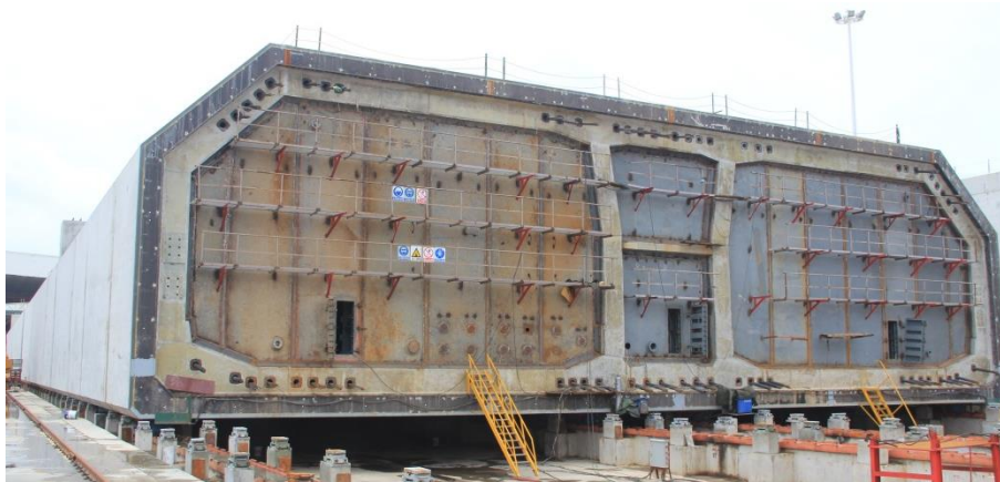
Figure 1. Segment of concrete tube tunnel in prefabrication of HZM project.
