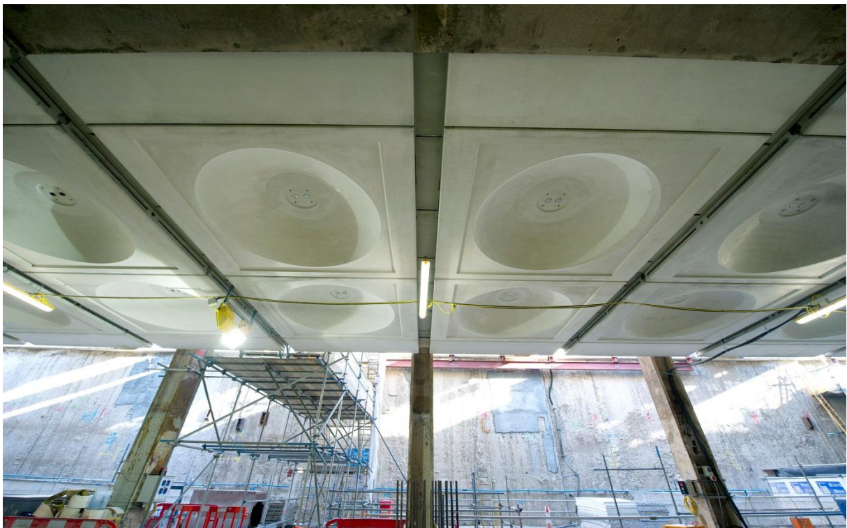
Figure 7: Exposed Coffers Slabs
