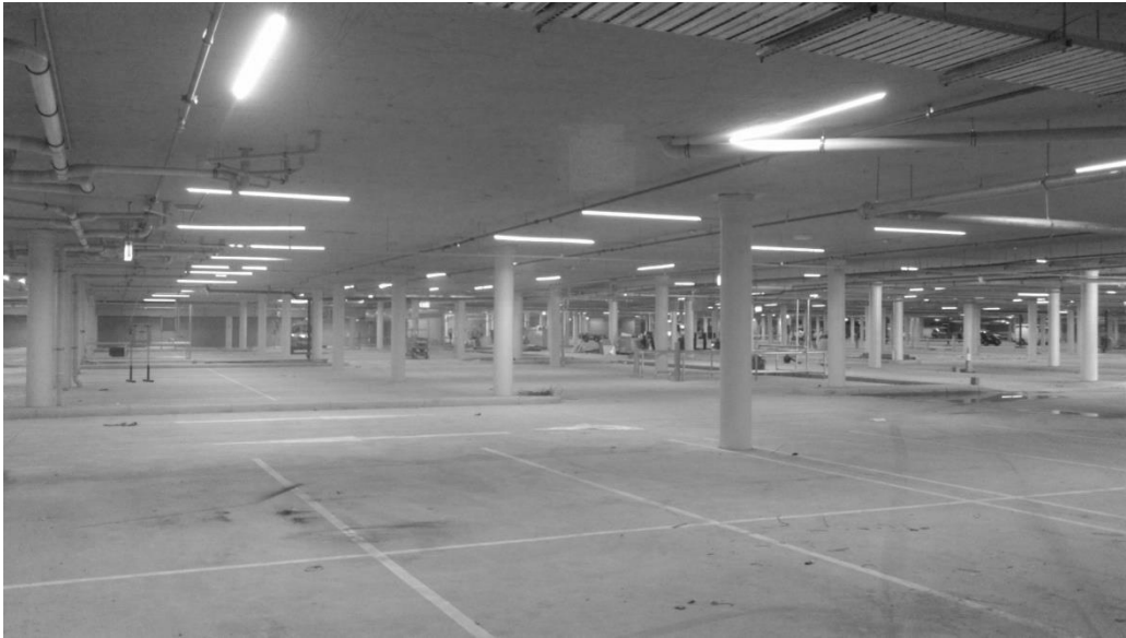
Figure 13. Photo illustrating the achieved verticality and alignment of the pile installation
