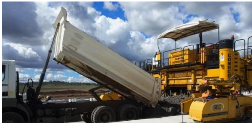
Figure 4. Geopolymer concrete delivery to slip form paver.
