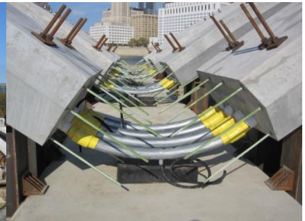
Close up view of the rib arches with post-tensioning ducts
