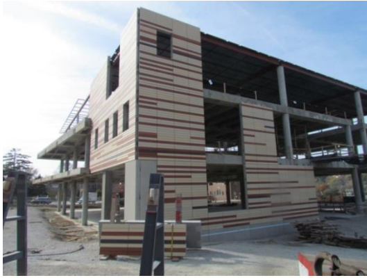
Erection of terracotta panels
