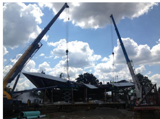
UHPC being installed on G8Way Pavilion
