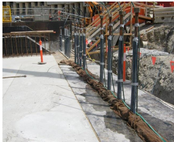
Figure 14. Forming and casting of concrete nib. Figure 15. Wet hessian applied on concrete nib.
