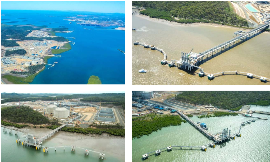
Figure 1. Top left: Overview of the Curtis Island LNG plants (from the bottom; Australia Pacific LNG, QCLNG and GLNG). Top right: GLNG. Bottom left: Australia Pacific LNG. Bottom right: QCLNG. @Bechtel
