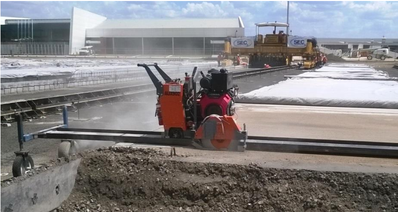
saw suspended on bridge to allow earlier joint formation
