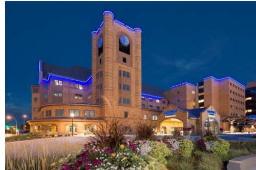
Finish perspective of thin brick cladding of Sanford Heart Hospital's clock tower
