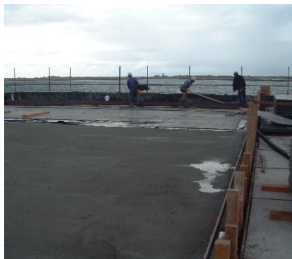
a) Insulation on a 2m Deep Jervoise Bay Deck
