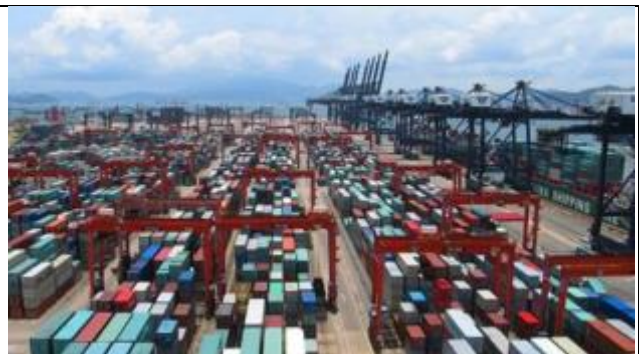
Figure 11. Completed container terminal
