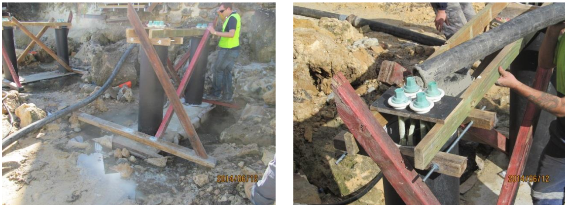
Figure 10. Forming and Pouring of Columns.
