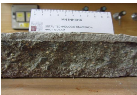
Figure 8. Fracture surface of mortar applied on the underlying concrete body
