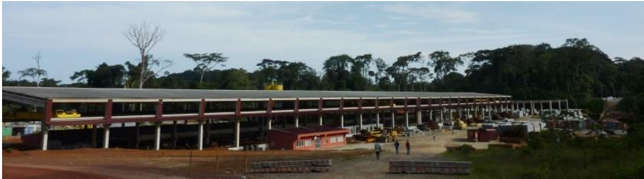
Figure 17. The 10,000 m 2 prefabrication plant in full operation
