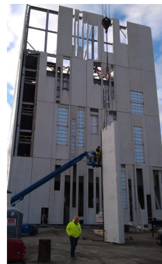
Erection of custom sized precast panels
