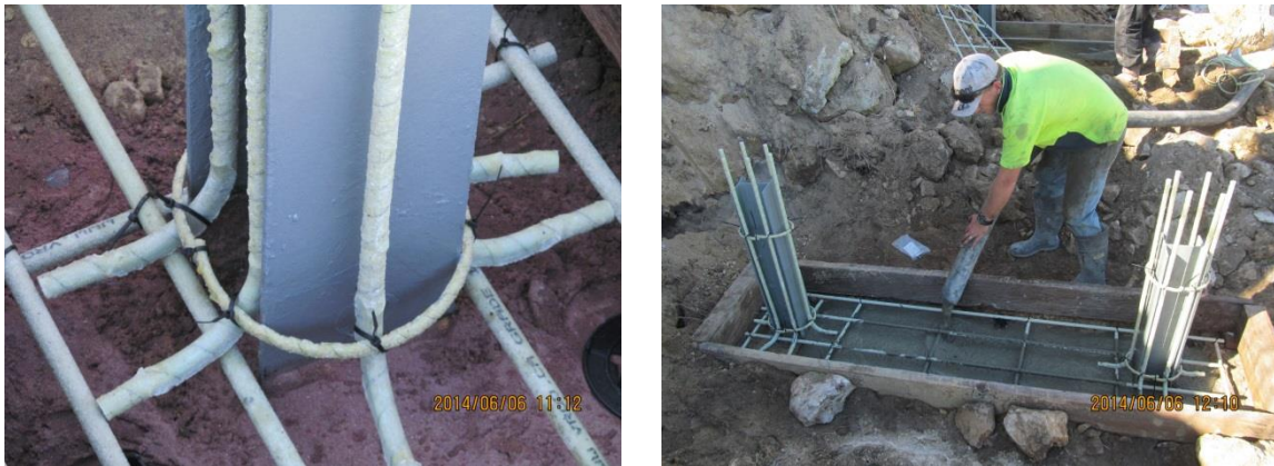
Figure 9. Forming and Pouring of Footings.
