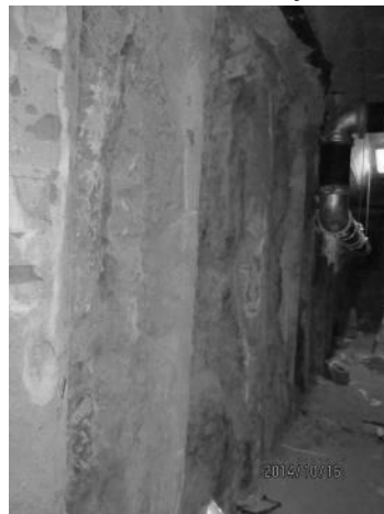
Figure 5. Detail of the free-draining cavity wall (left); Constructed air-shaft and soil retaining (right)
