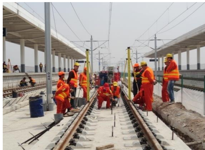
Figure 4. Grouting quick uplifting rehabilitation construction of Yongji North Station on site.
