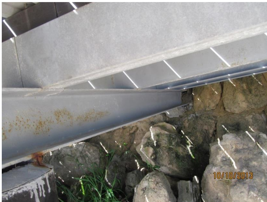
Figure 4. Steel Cross Beam Embedded in Retaining Wall.
