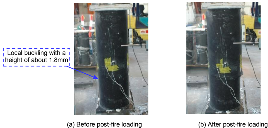
Figure 7. Failure mode of CFST-03.
