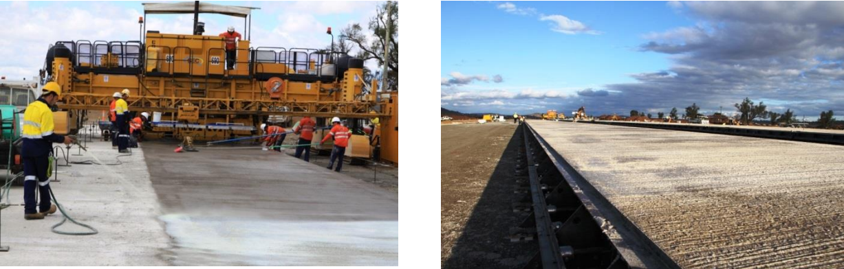
Figure 6. Curing and side forms with dowels.
