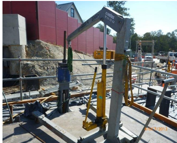
Figure 18. Stress bar stressing arrangement.
