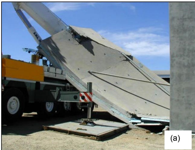
Figure 3. 35 tonnes panel that collapsed onto a crane during erection (WorkSafe Victoria, 4): (a) photo of collapsed panel; b) photo of a failed coil anchor used as a bracing insert.
