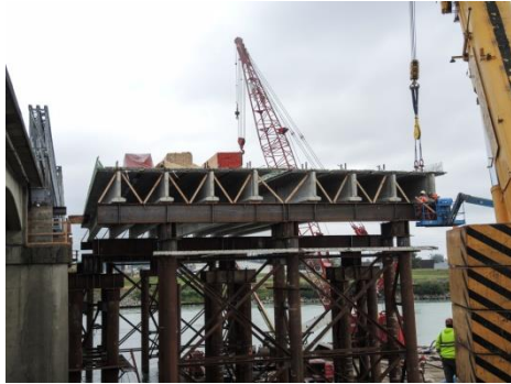
Rehabilitation of New York Avenue bridge Permanent concrete girder system
