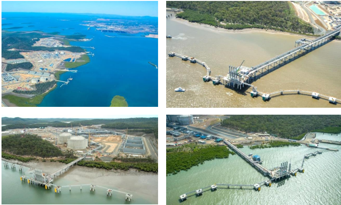
Figure 1. Top left: Overview of the Curtis Island LNG plants (from the bottom; Australia Pacific LNG, QCLNG and GLNG). Top right: GLNG. Bottom left: Australia Pacific LNG. Bottom right: QCLNG. ©Bechtel
