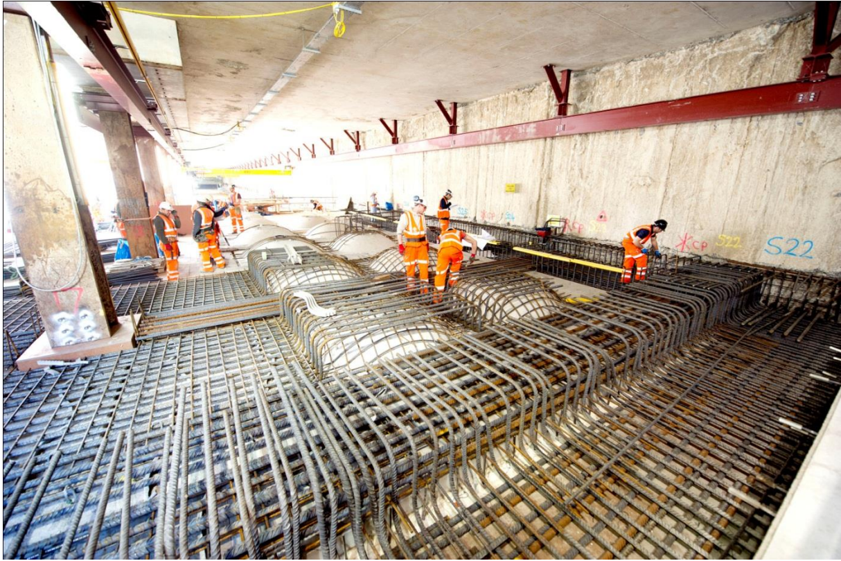
Figure 6: Structural slab reinforcement being fixed on precast concrete ceiling panels
