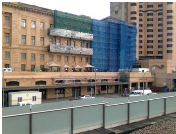
Figure 4. First of 3 stages of scaffolding for the Northern Façade conservation works.
