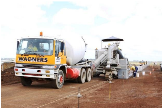
Figure 9. Other Geopolymer Concrete Works at BWWA.
