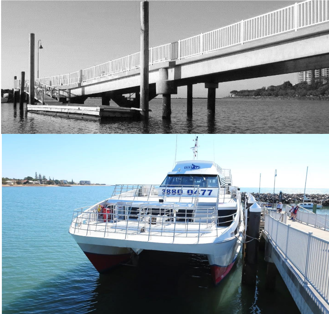
Figure 7. Top: Southern Finger. Bottom: Northern Finger with Commercial Tour Operator Vessel (note the independent fender piles). @Arup
