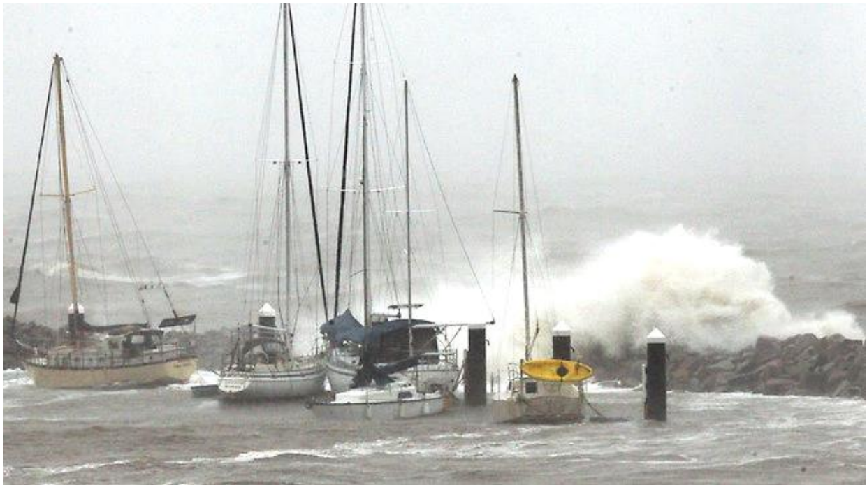
Figure 6. Redcliffe Jetty Breakwater During January 2013 Storm Event. @Arup
