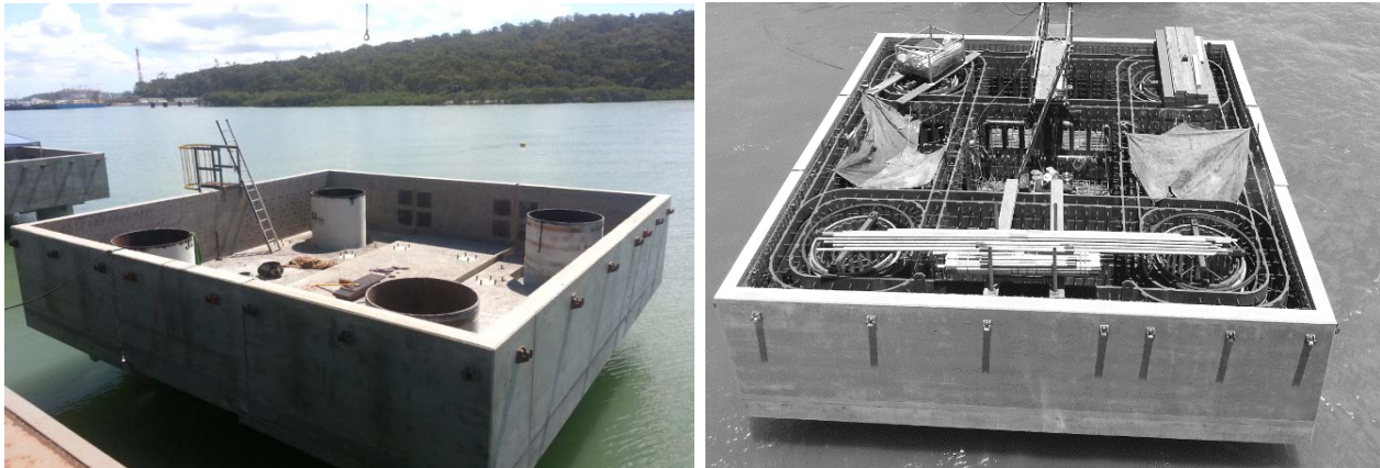
Figure 10. Precast Berthing Dolphin Shell before and After Reinforcement Installation. @Arup
