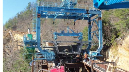
Segments of precast being placed
