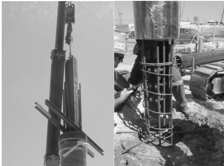
Figure 7. Caisson lifting and cage splicing
