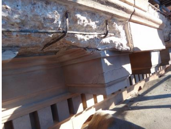
Figure 5 – Removal of defective concrete along the edge of the top ledge
