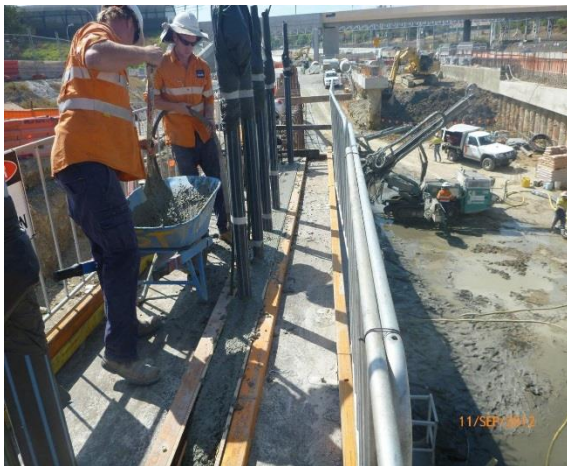
Figure 14. Forming and casting of concrete nib. Figure 15. Wet hessian applied on concrete nib.
