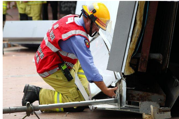
(b) End of awning with anchors showing.
