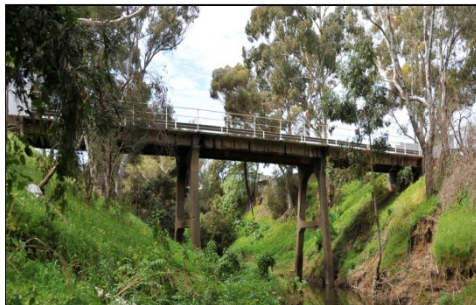
Figure 2 The bridge prior to restoration
