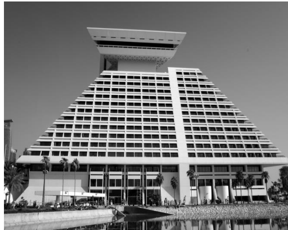
Photo 11: Renovated Hotel Sheraton Doha right side view. ( Sea water inlet in the front side)
