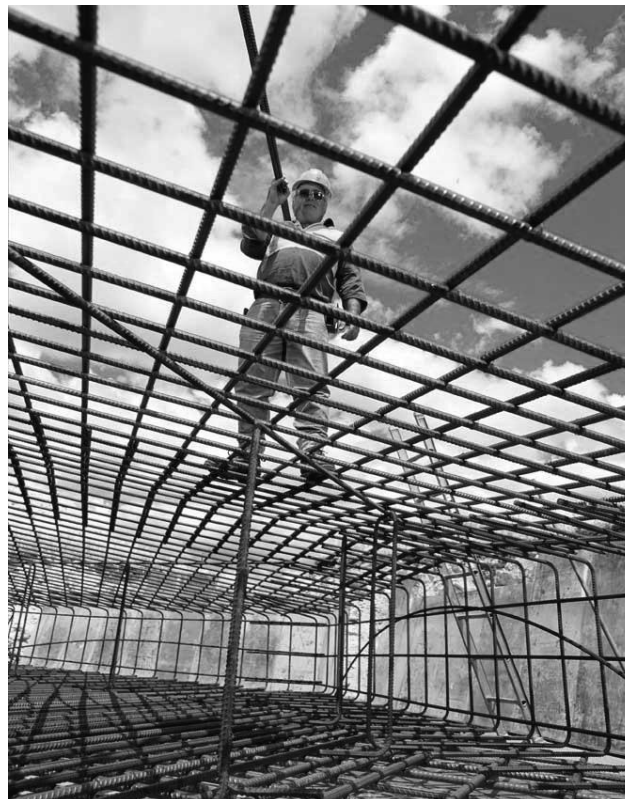
Figure 2. Top steel supported from bottom steel using “engineer specified” supports.
