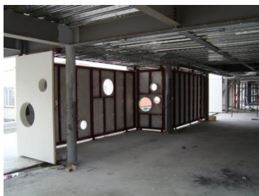
Precast panel wall installation
