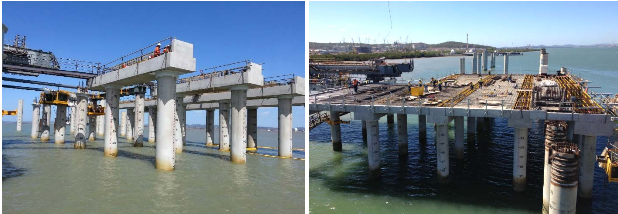
Figure 8. Australia Pacific LNG Jetty Loading Platform during Construction. @Arup
