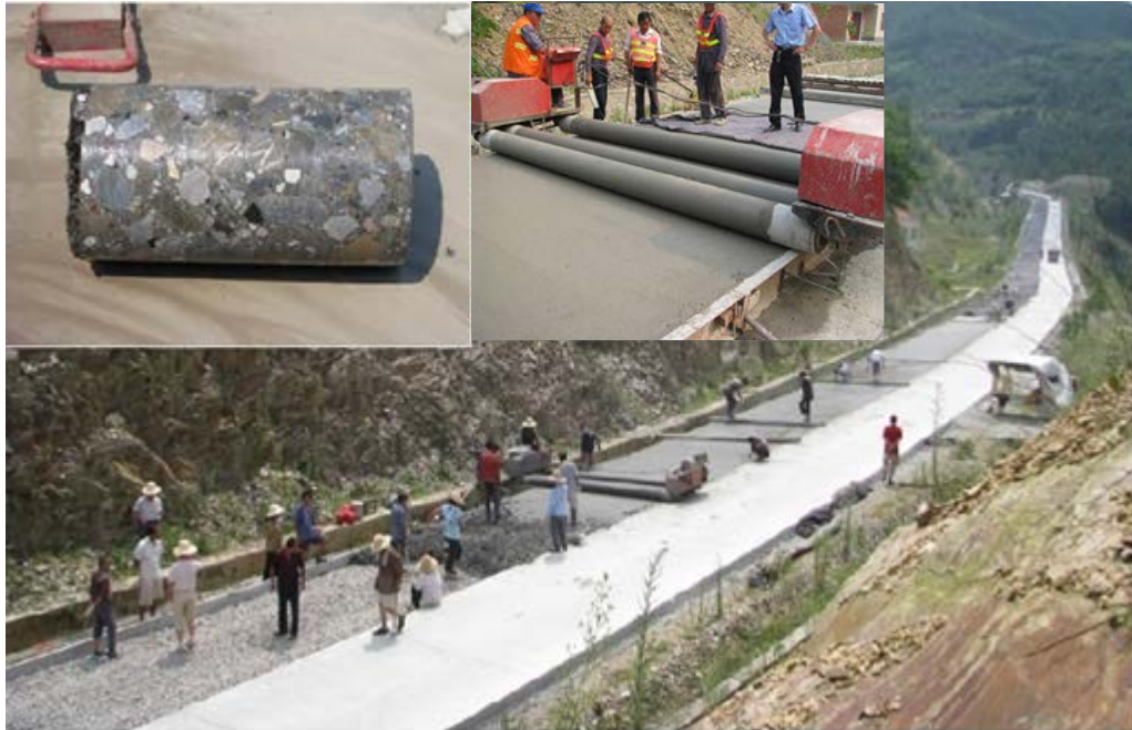
Figure 4. The building site of SFSC pavement
