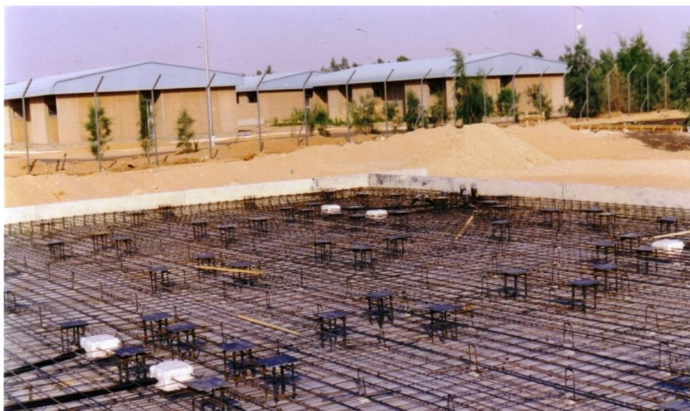
Figure 8. Finished houses, and a foundation raft for an additional one
