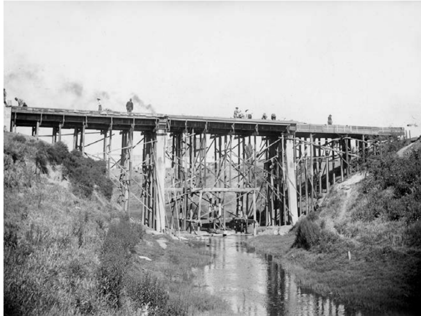
Figure 1 The bridge under construction 1908
