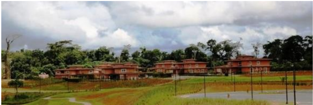
Figure 15. One group of the villas, built with precast concrete panels,
