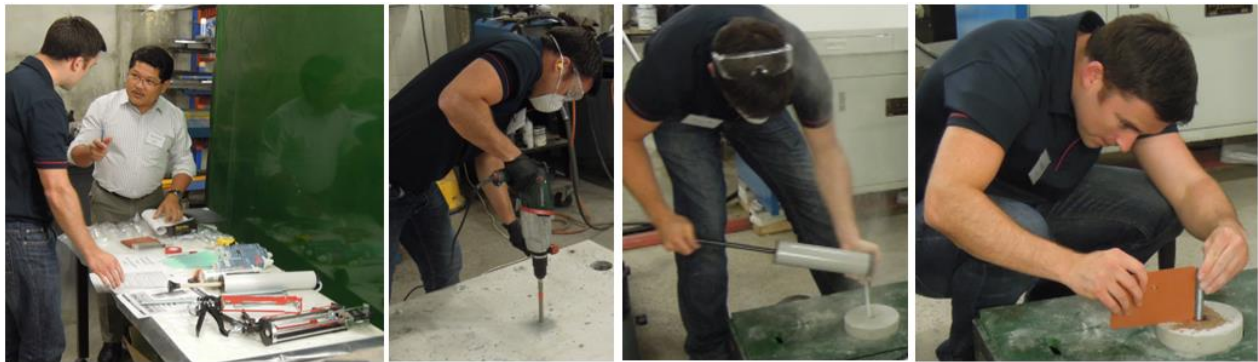
Figure 15. Vertical down bonded anchor installation
