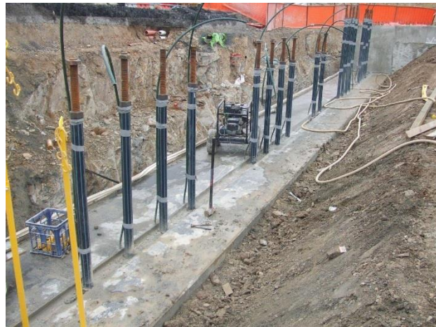
Figure 13. Completion of stage 1 works.
