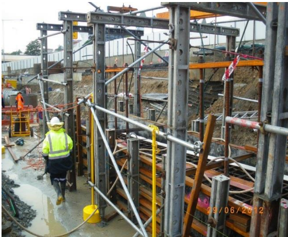
Figure 12. Stress bars supported by scaffolding system.
