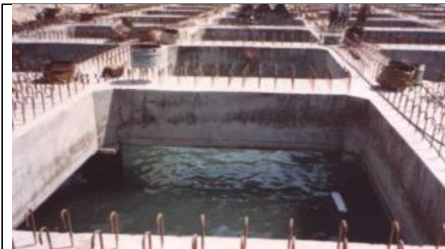
Figure 10. Foundation coated with cementitious coating
