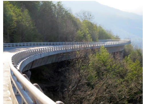
Foothills Parkway Bridge Completed
