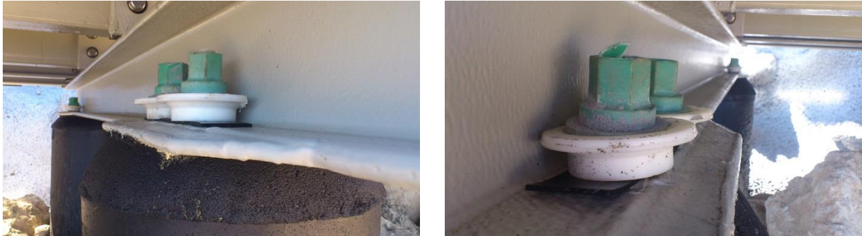
Figure 11. Column and Steel Connection.
