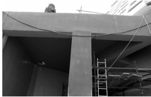
Photo 6: The beam and column of seawater intake structure after repair work
