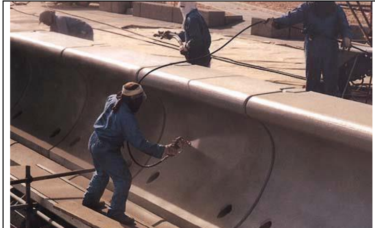
Figure 12. Application of cementitious coating system
