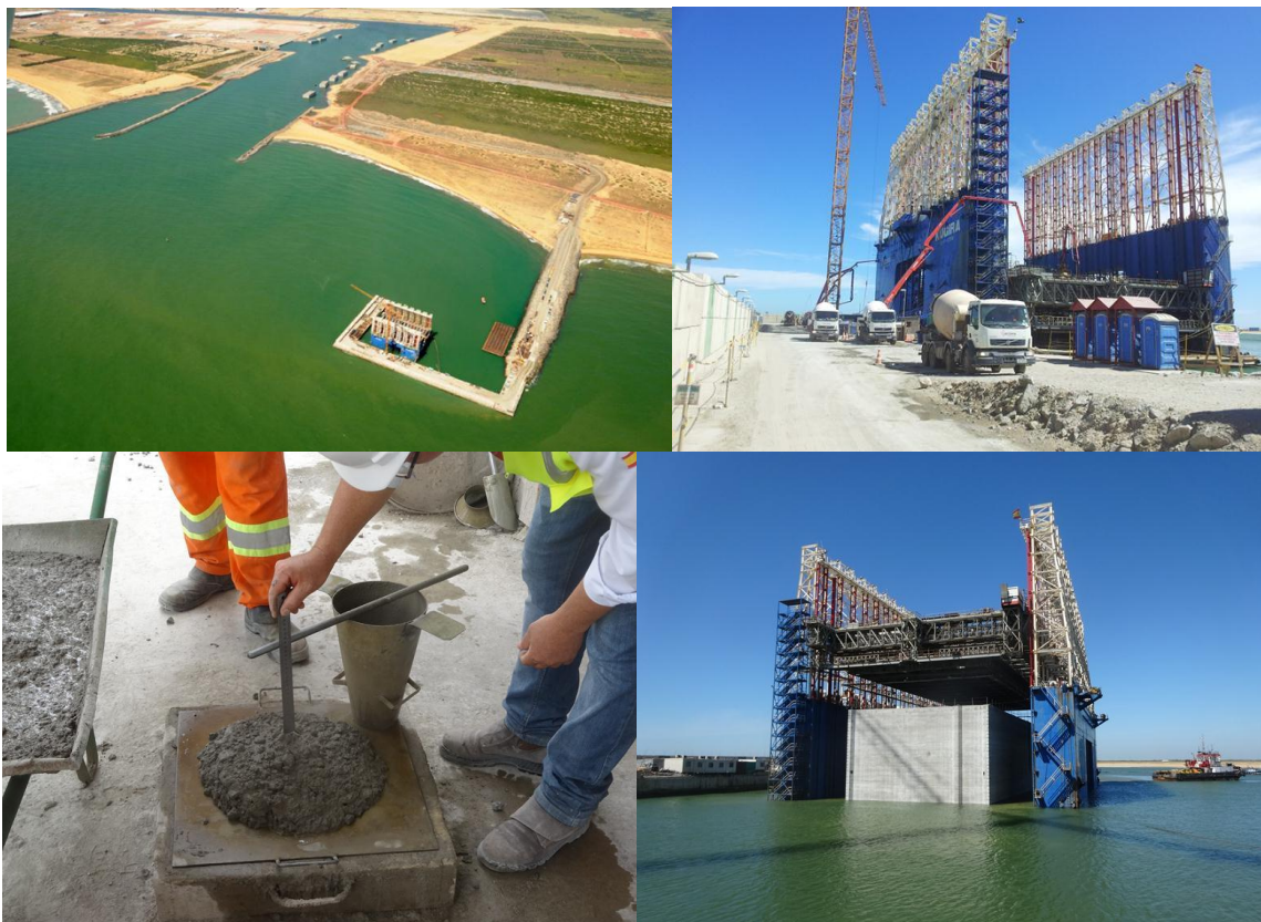
Figure 8. Work site pictures. Provisional Kugira protective dock, Kugira and 22 cm slump
