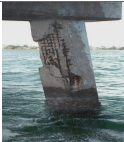
Figure 2. Result of Chloride attack on concrete Jetty
