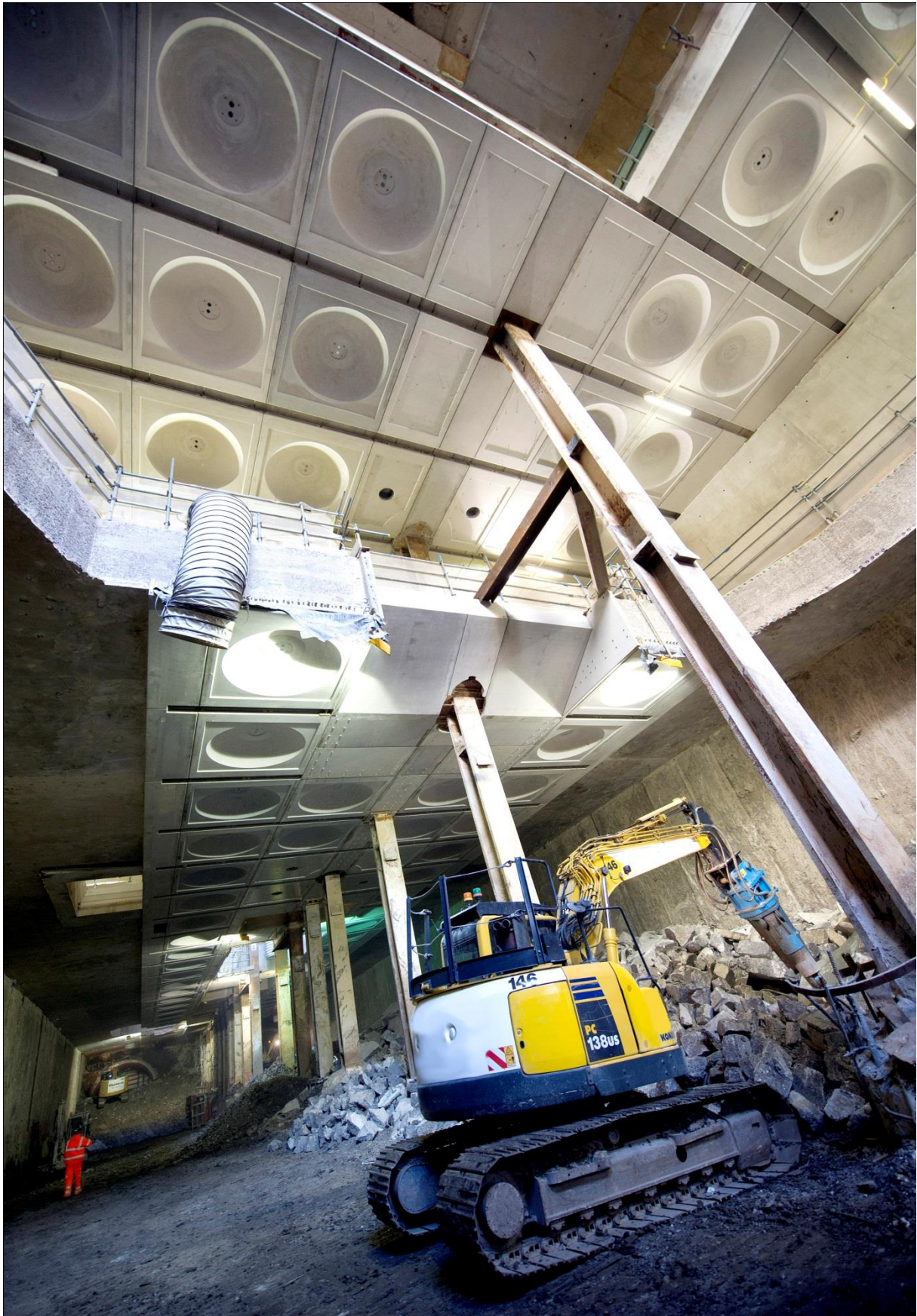
Figure 8: Exposed platform ceiling (Note temporary steel piles penetrating the concrete ceiling)
