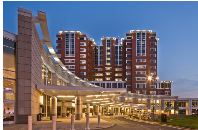
Finished perspective of The University of Kentucky Albert B. Chandler Hospital Pavilion
