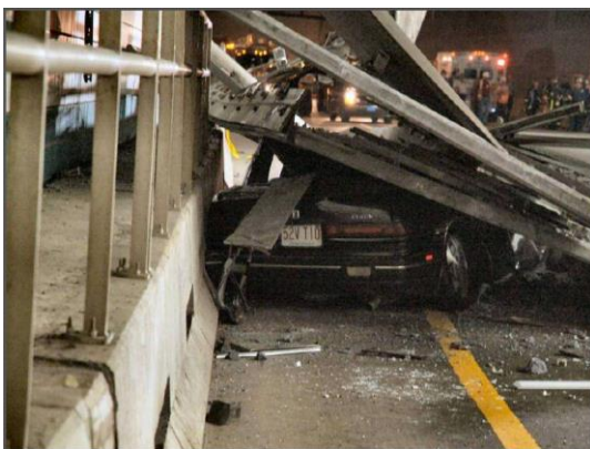
Figure 2. Concrete ceiling tiles collapse in the Big Dig Tunnel, 2006: (a) photo of aftermath; (b) photo of roof hangers pulled away from tunnel roof (Brady,3).
