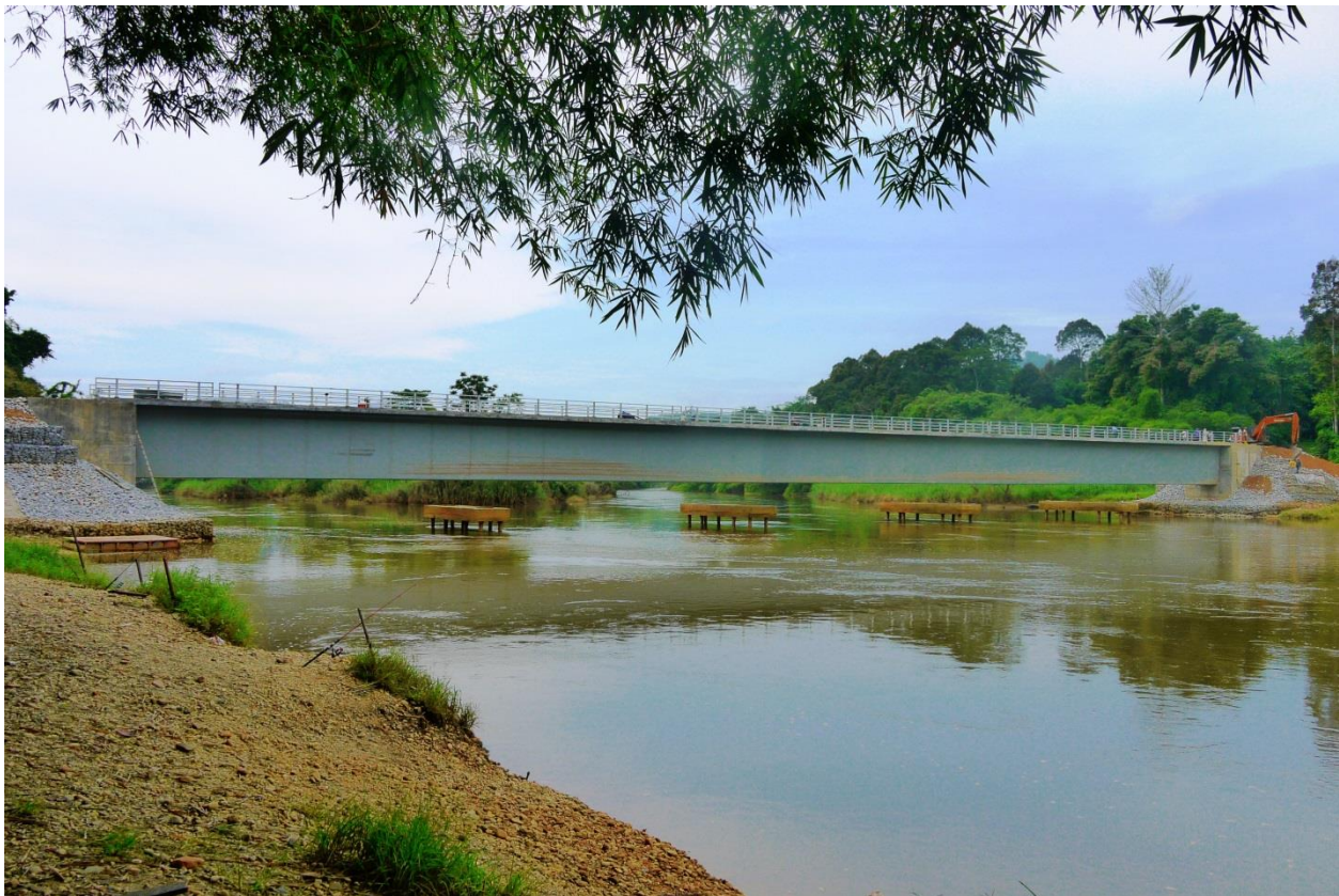
Figure 8. 100 metre span Batu 6 Bridge – completed May 2015.
