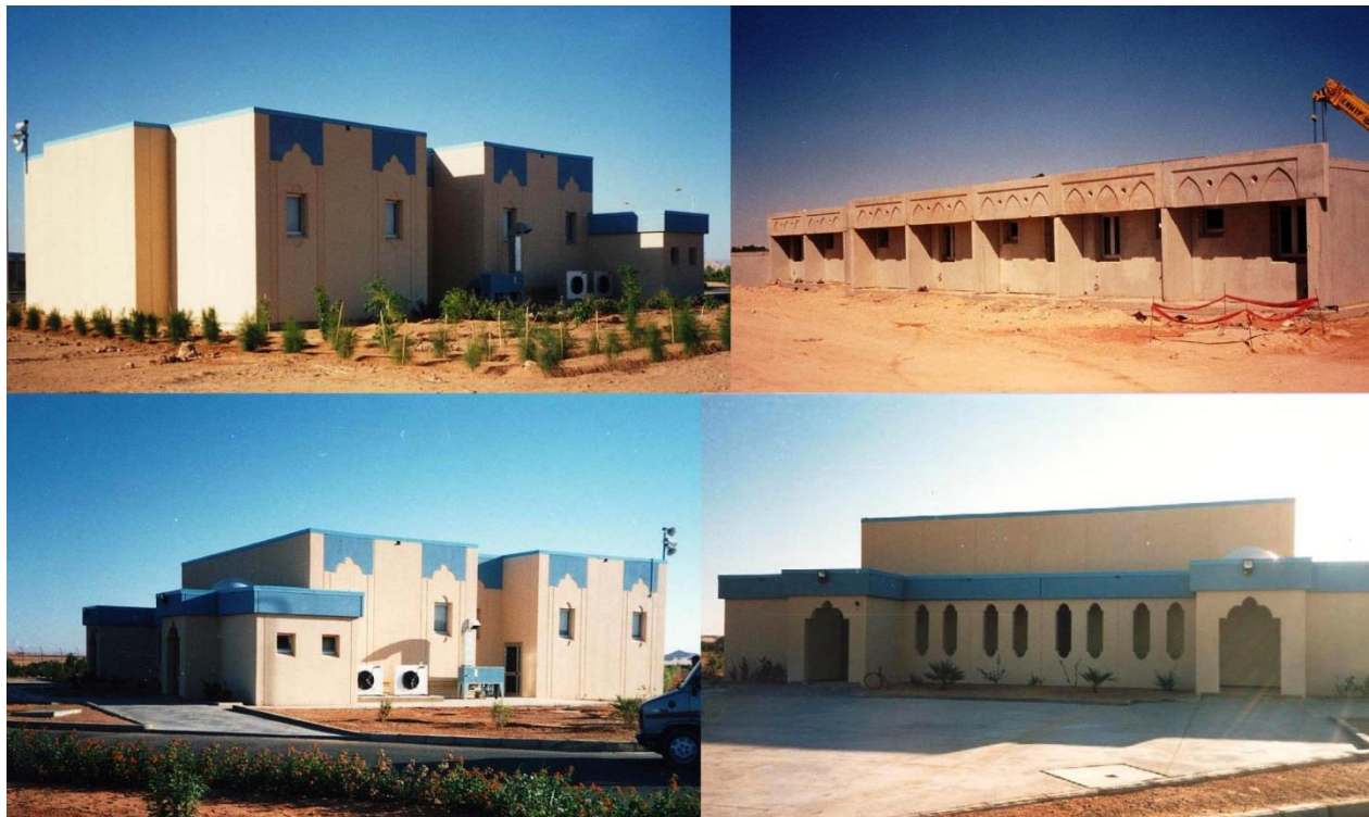
Figure 10. Examples of houses built with cellular concrete precast wall panels
