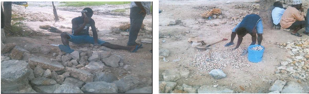
Figure 1: Local people crushing big concrete debris to aggregate sizes
