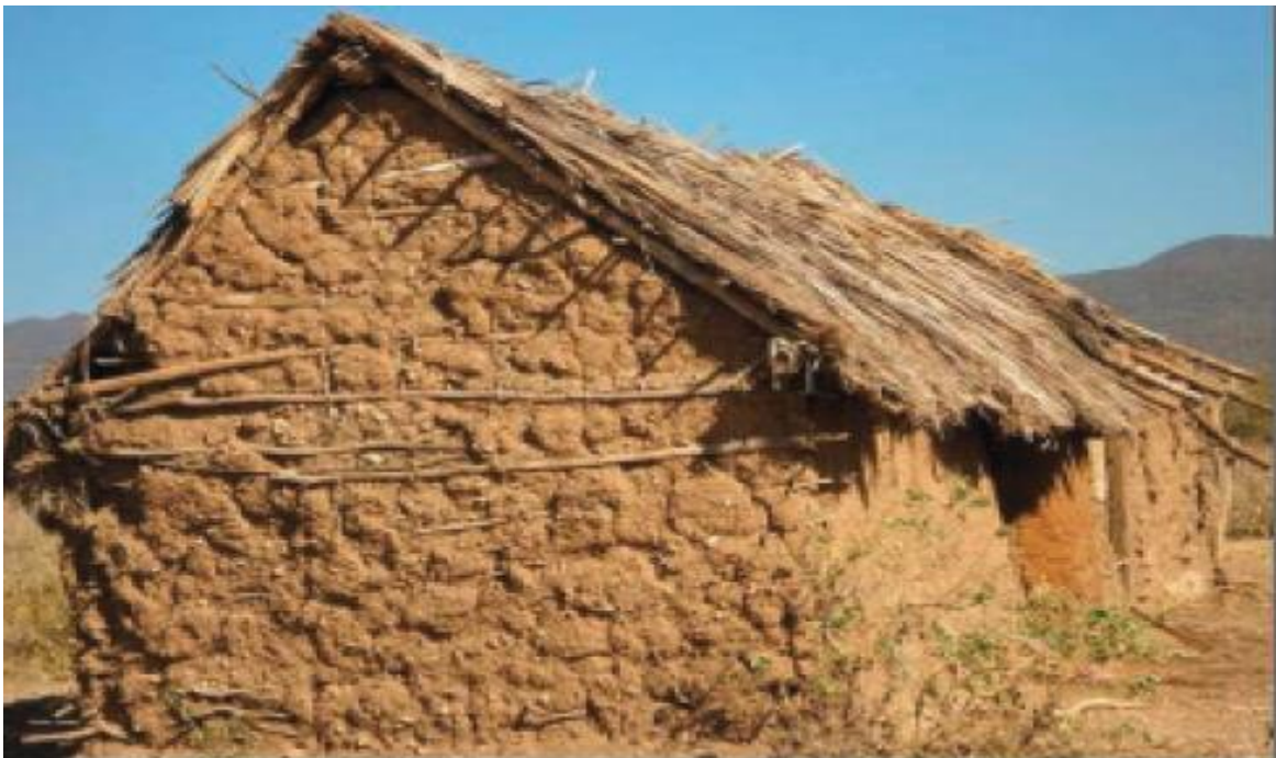
Figure 1: Earth Construction (Courtesy J. Makunza)
